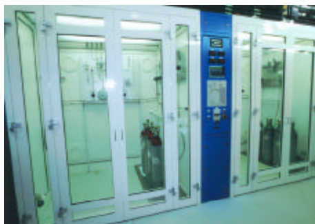
New corrosive filling workshops
